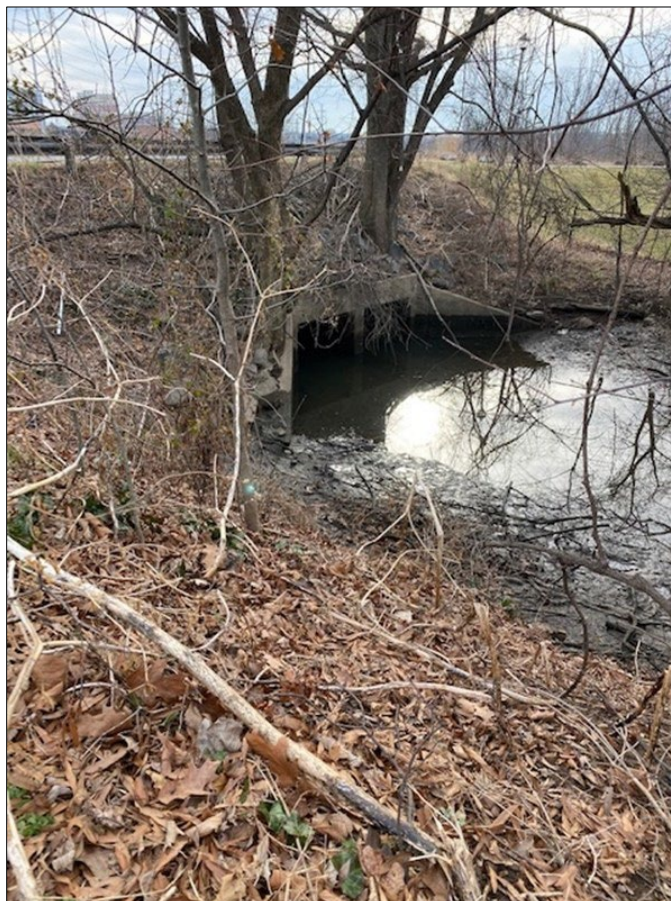
Figure 4-6. Existing Culvert Crossing in the Location of the Proposed Culvert Crossing at the West Stream in Four Mile Run
