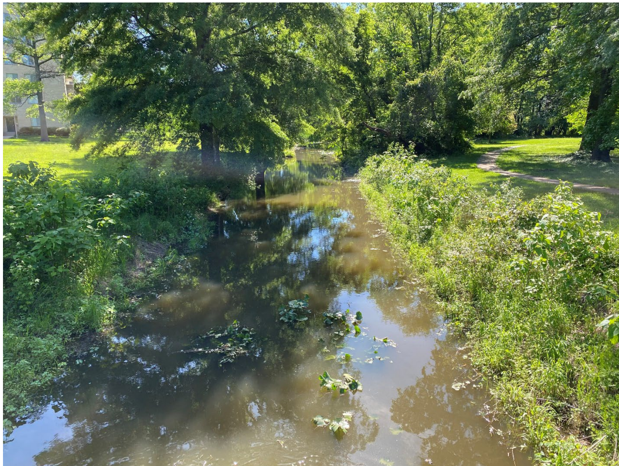
Figure 4-8. Location of the proposed culvert crossing at the Belle Haven West Channel
