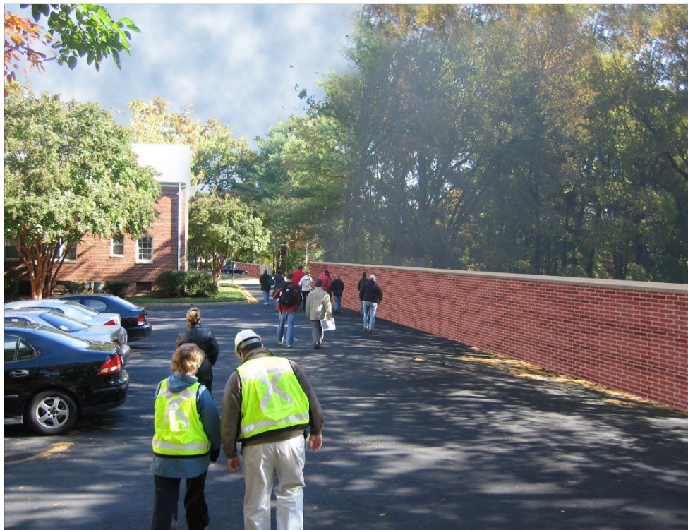
Figure 4-10. Rendering of a 6.5-ft Floodwall South of the River View Condominiums Located at Boulevard View and 10 th Street
