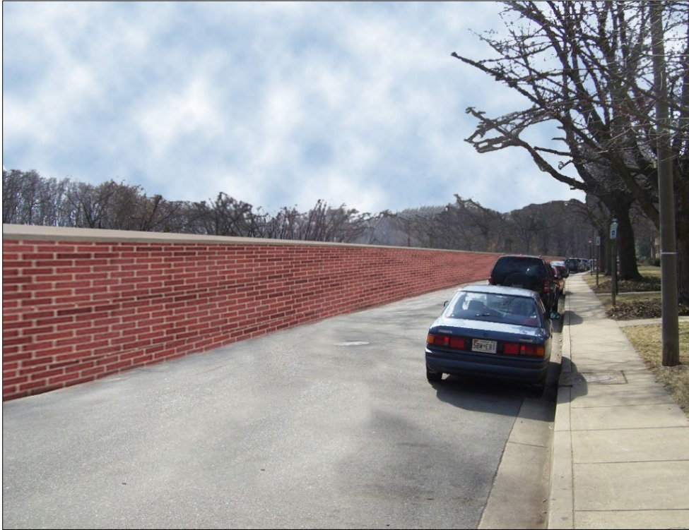
Figure 4-9. Rendering of a 6.5-ft-tall Floodwall Along the East Side of Boulevard View
